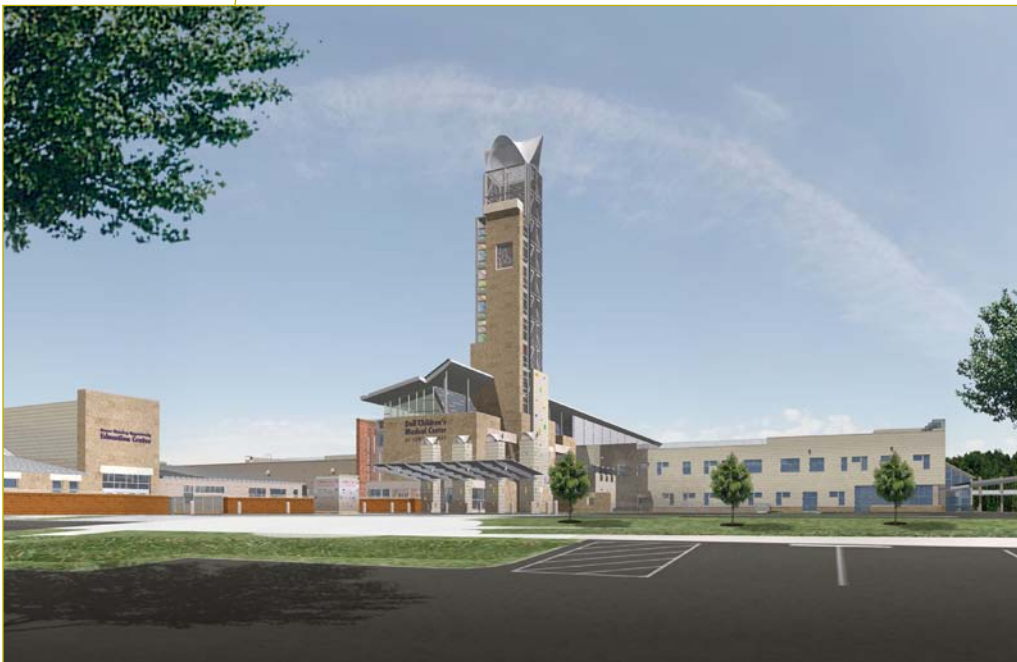
Proposed Main Entry, Dell Children's Medical Center of Central Texas Austin, TX
